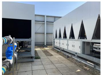
Critical heating and cooling infrastructure upgrades for the University of York Biology Block including the replacement 2no. 750kW chillers, 1no. 450kW chiller, 4no. 750kW boilers, associated hot & chiller water pipework as well as primary and secondary pump sets.
